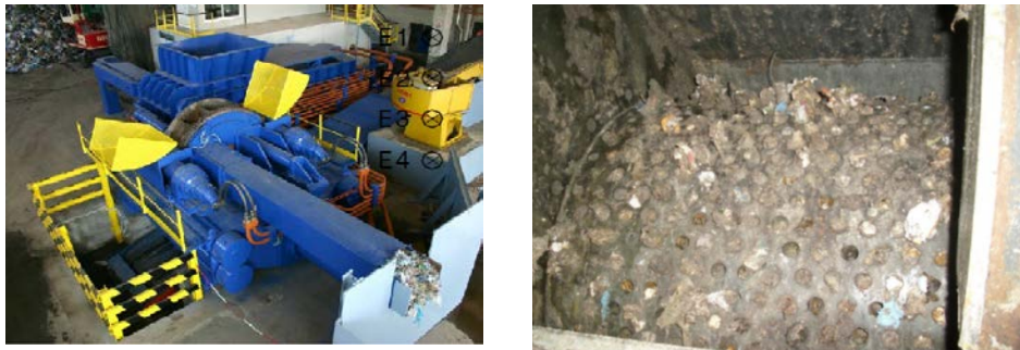
Picture 6. „Waste sorting and recycling facility in Ventspils MWM region”
