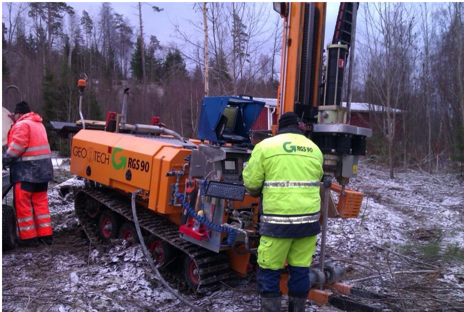
Figure 3: Direct push injection rig on site
