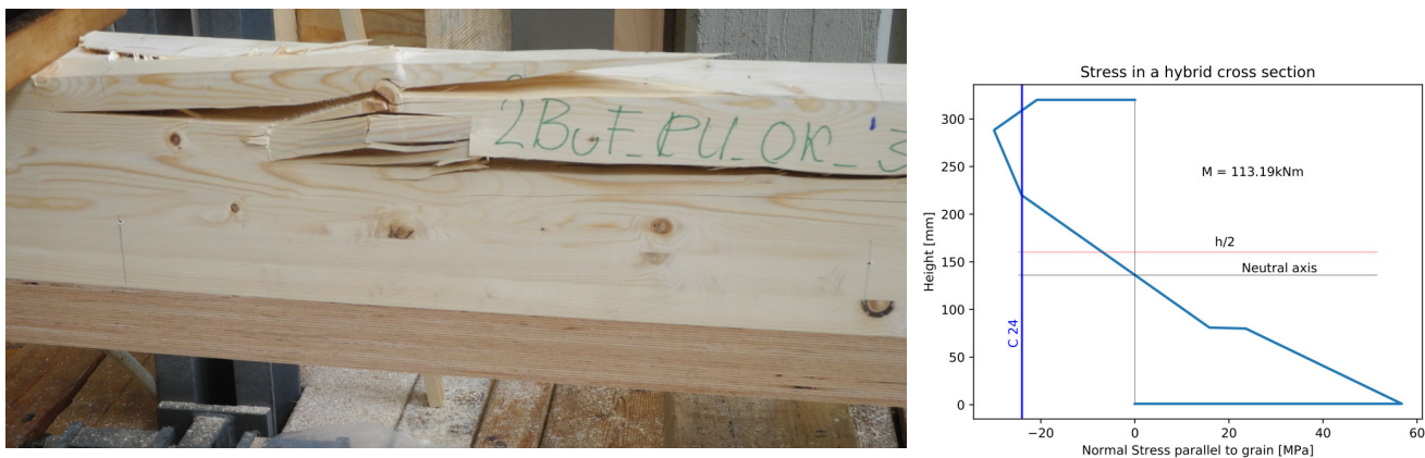
Figure 1: GLT beam with 25 % Beech LVL Reinforcement
